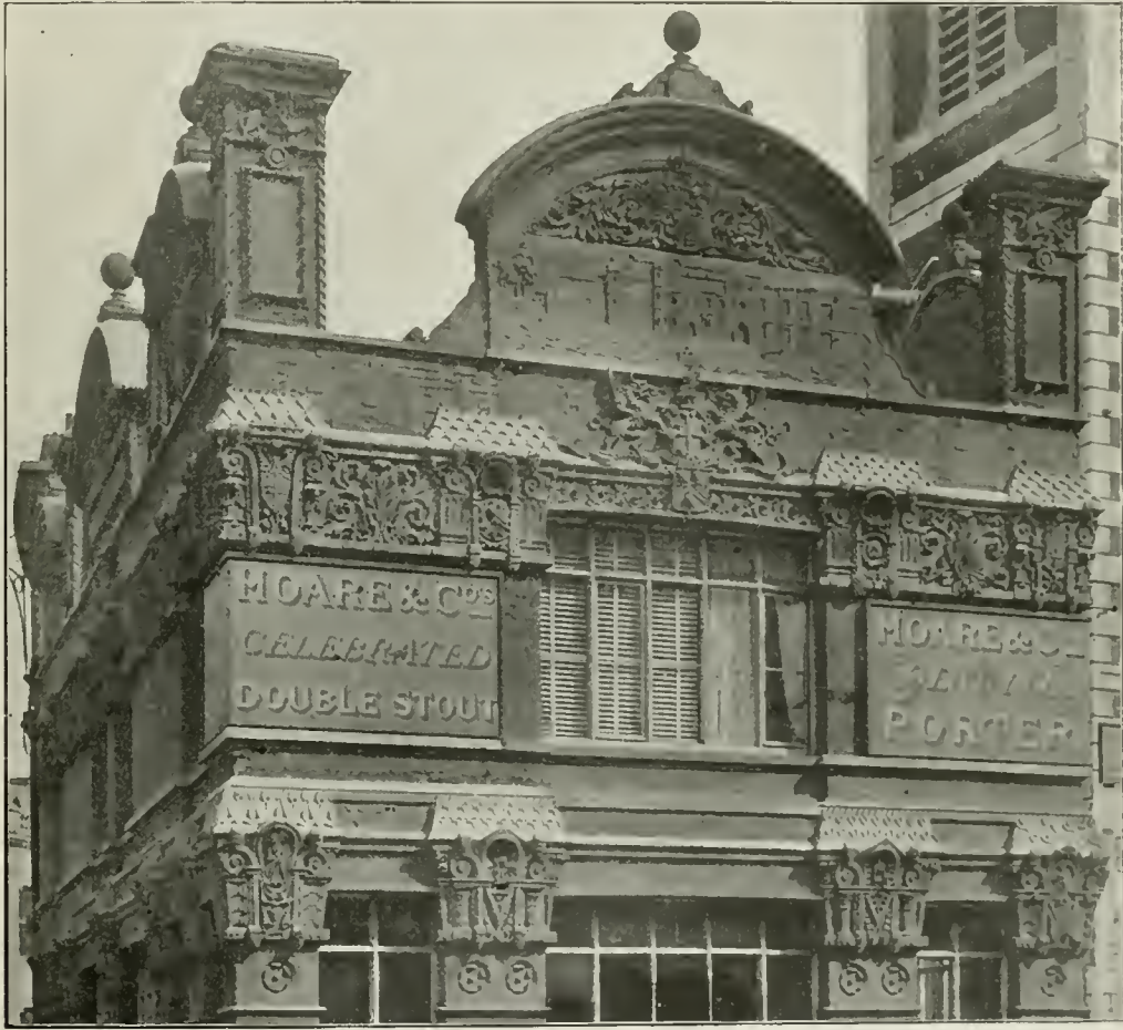
No. 78.—EXTERIOR ORNAMENTATION IN PORTLAND CEMENT, MODELLED in situ BY W. MILLAR, 1874. BAYNARD CASTLE HOTEL, LONDON.
